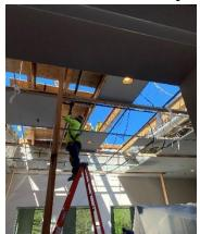
Damaged roof joists and plywood have been replaced - the new TPO roofing membrane is installed. And the parking lot is empty of roofing material!
