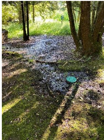
This is the area behind B3 before installation of the bioswale. The green valve box is where the pumped water flowed out of the garage and onto the surface
