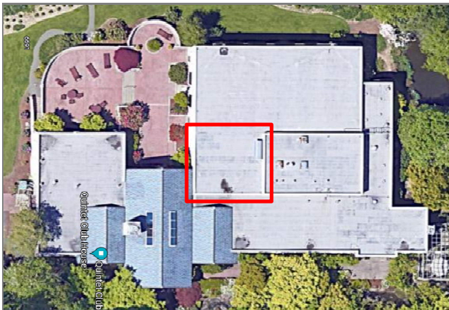
Quintet Clubhouse Roof (Image from Google Maps)
