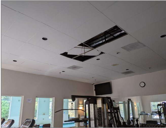
Figure 13 Drop ceiling at exercise room.
