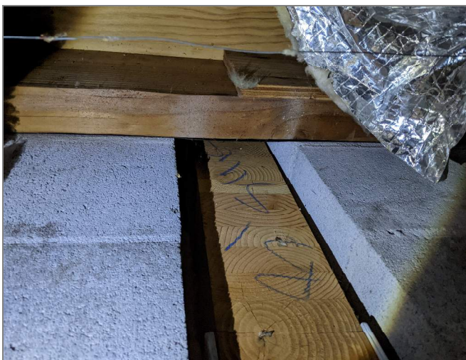
Figure 15 Glulam beams bearing in CMU wall.
