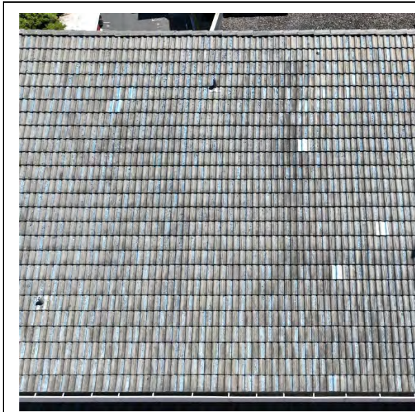
Typical steep slope tile roof.
