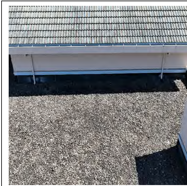
Typical low slope EPDM roof with ballast river rock.
