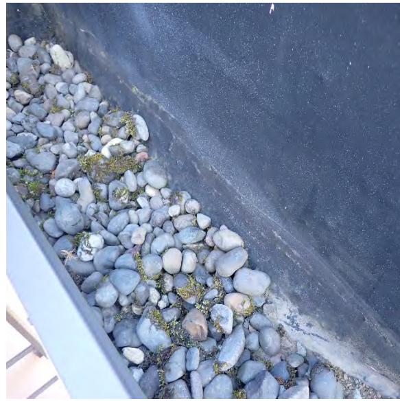
Typical EPDM wall flashing.
