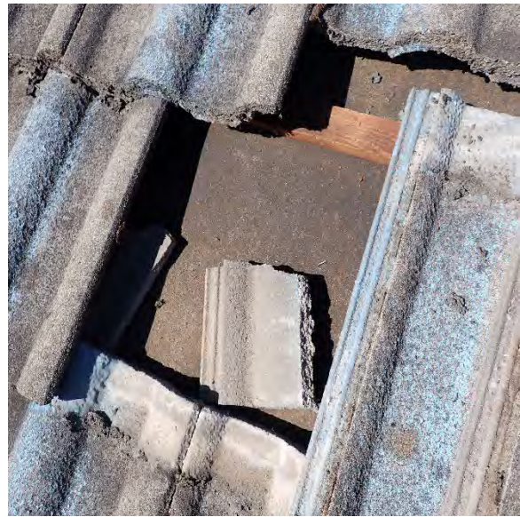
Typical underlayment used for tile roofs.
