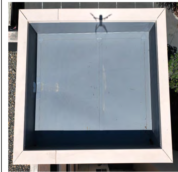
Typical new low slope PVC single ply roof above stairways.
