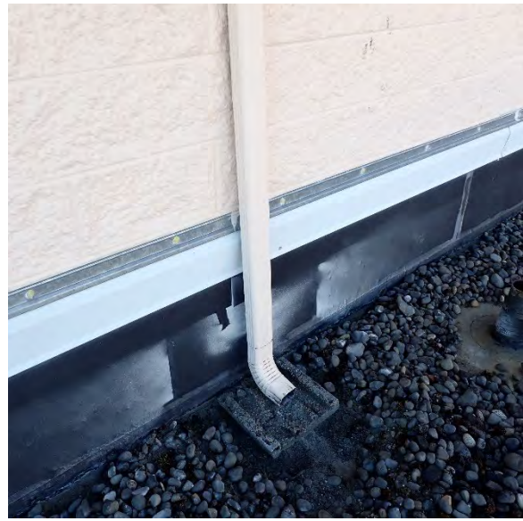
1.10 Typical downspout with splash block.
