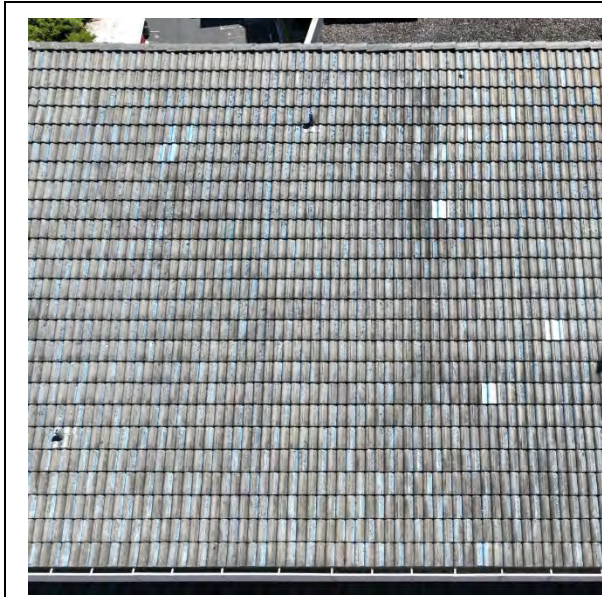
1.1 Typical steep slope tile roof.
