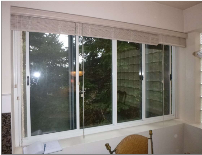
Figure 3.26 Typical 4-pane sliding window.
