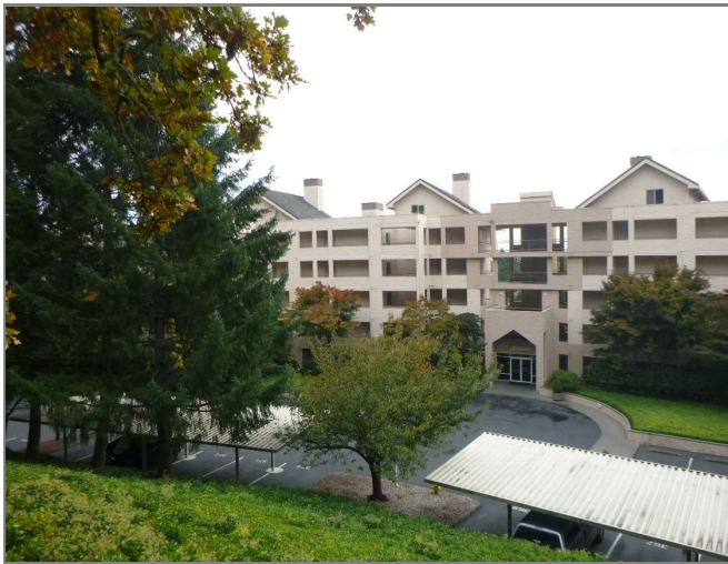
Figure 2.1 North elevation at Building 4
