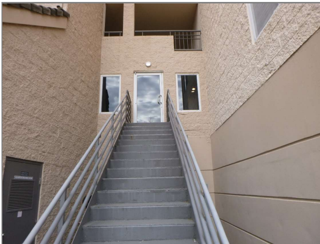
Figure 3.44 Rear door at central elevator lobby
