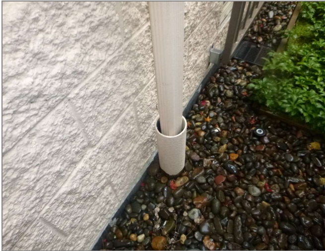
Figure 3.89 Building 1 Downspout drains into PVC pipe that extends below raised planter
