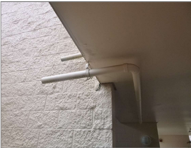
Figure 3.75 Building 1 Drain pipe at underside of floor in Figure 3.73
