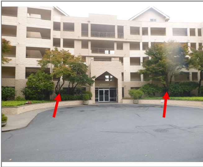
Figure 3.113 Building 4 Large established trees growing in center front planters
