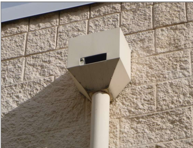
Figure 3.98 Clubhouse Typical scupper box with overflow.
