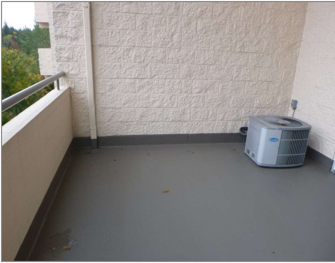
Figure 3.58 Unit 340 Typical residential unit balcony
