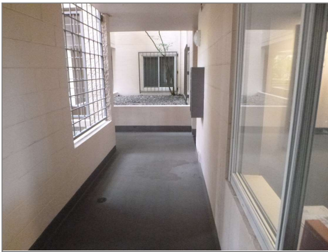
Figure 3.66 Building 5 Typical ground floor open-air corridor.
