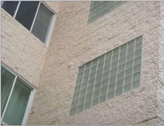
Figure 3.18 Glass block inserts, typical
