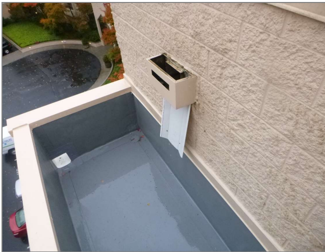
Figure 3.76 New roofing installation in-progress at Building 4
