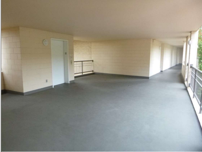
Figure 3.70 Building 5 Typical open-air corridor at elevator lobby.
