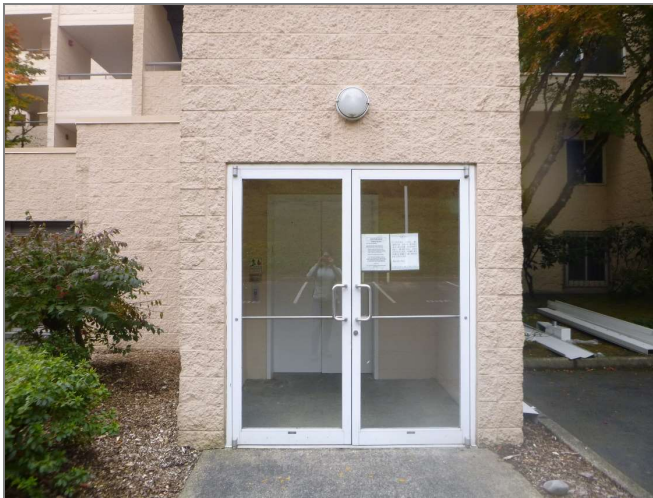
Figure 3.43 Building 4 Typical auxiliary elevator lobby storefront door.
