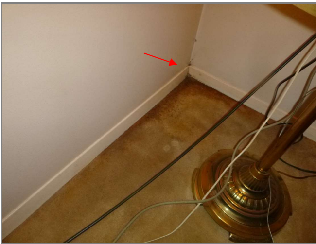
Figure 3.4 Unit 111 Elevated moisture content and potential organic growth at NW corner of second bedroom.
