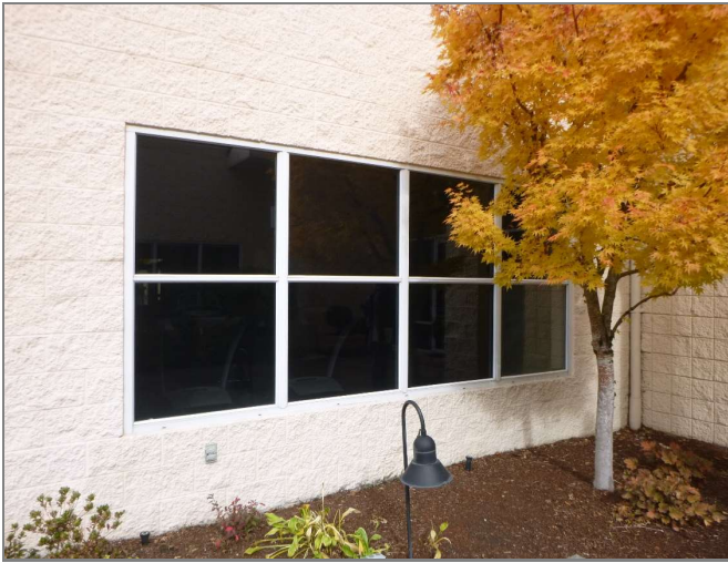
Figure 3.29 Clubhouse south elevation 8-pane fixed windows.
