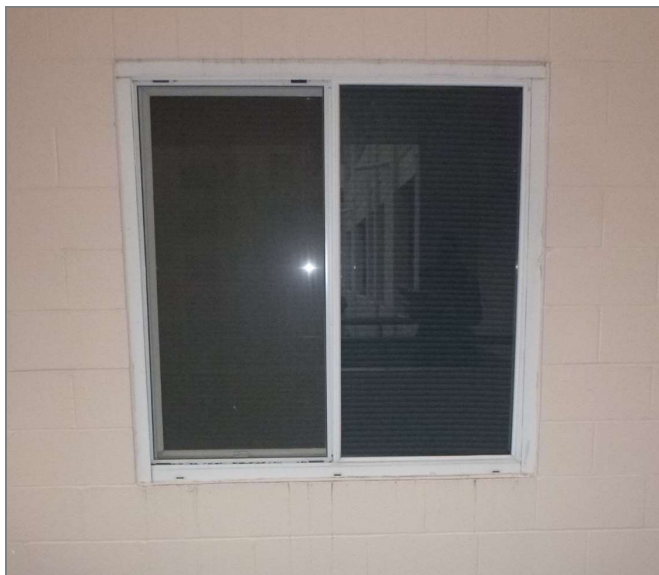
Figure 3.25 Building 2 corridor Typical 2-pane sliding window.
