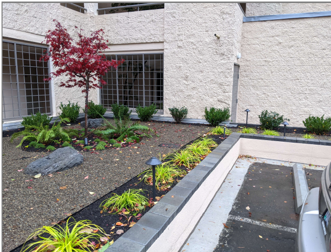
Figure 3.109 Building 1 Renewed planter with coated CIP concrete wall
