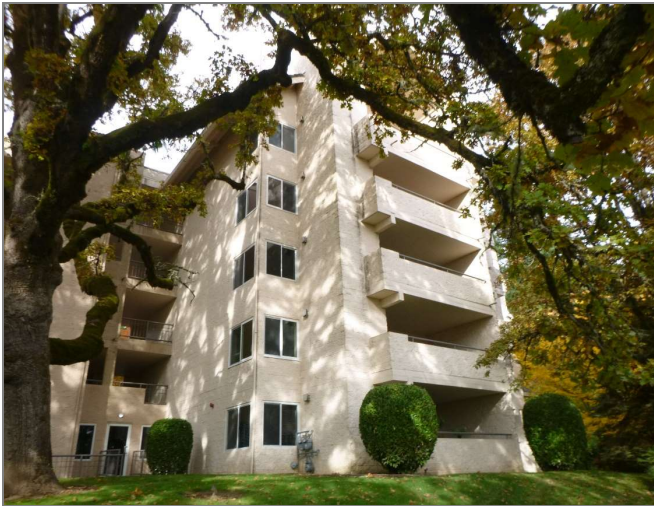
Figure 2.2 Southeast elevation at Building 5
