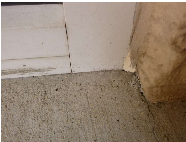
Figure 3.47 Clubhouse west elevation Hardscape covers bottom edge of storefront system.
