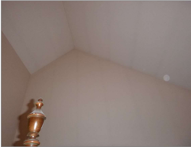
Figure 3.1 Unit 520 "Stud shadowing" at vaulted ceiling
