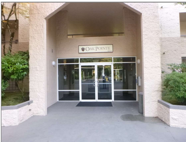
Figure 3.41 Building 5 Storefront system at building entry.
