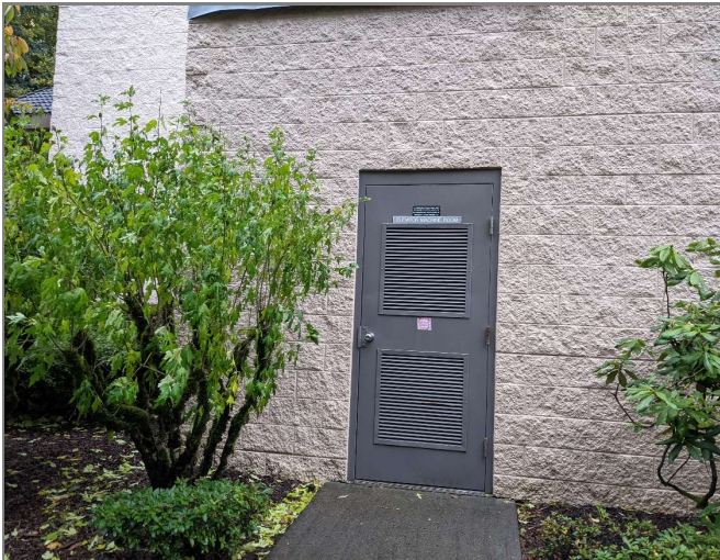
Figure 3.52 Building 1 Typical elevator machine room door.
