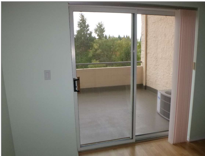
Figure 3.35 Unit 340 Typical sliding door.
