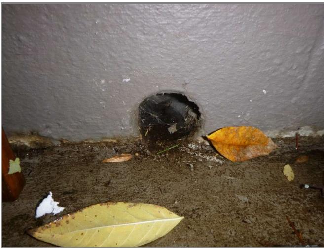
Figure 3.60 Unit 216 Typical round scupper.
