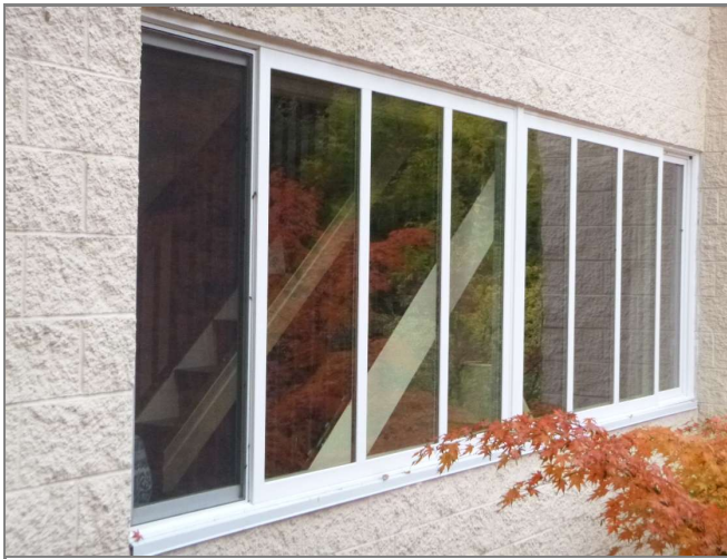
Figure 3.27 8-pane sliding window. Example has been replaced with new vinyl-framed system.
