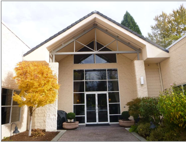
Figure 3.42 Clubhouse west elevation Storefront system at clubhouse atrium
