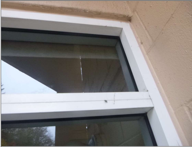
Figure 3.45 Building 1 Typical storefront gasket, mullions, and perimeter seal.
